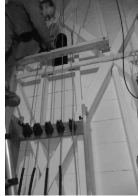
Neil Thomas of Whitechapel Bell Foundry working on the installation
